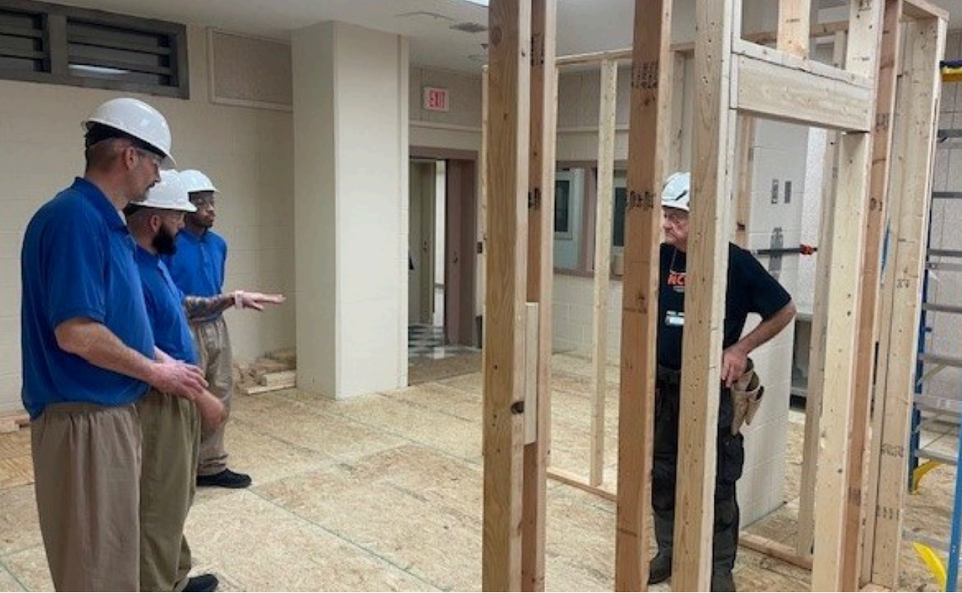
Participants ask questions during construction-related job training. Photo Credit: MCSO
